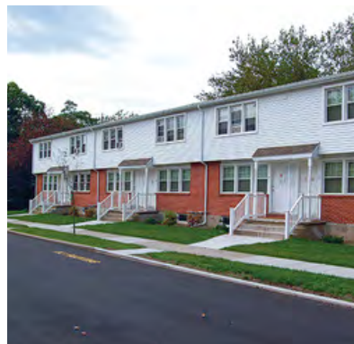
Savin Court Apartments
